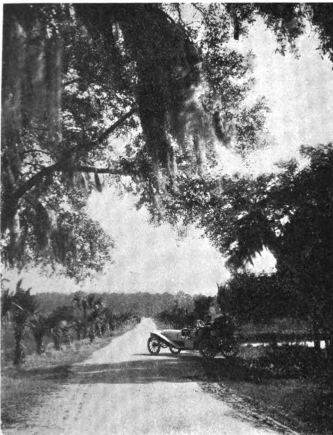
ONE OF THE BEST STRETCHES ON LA ROCHE AVENUE.
